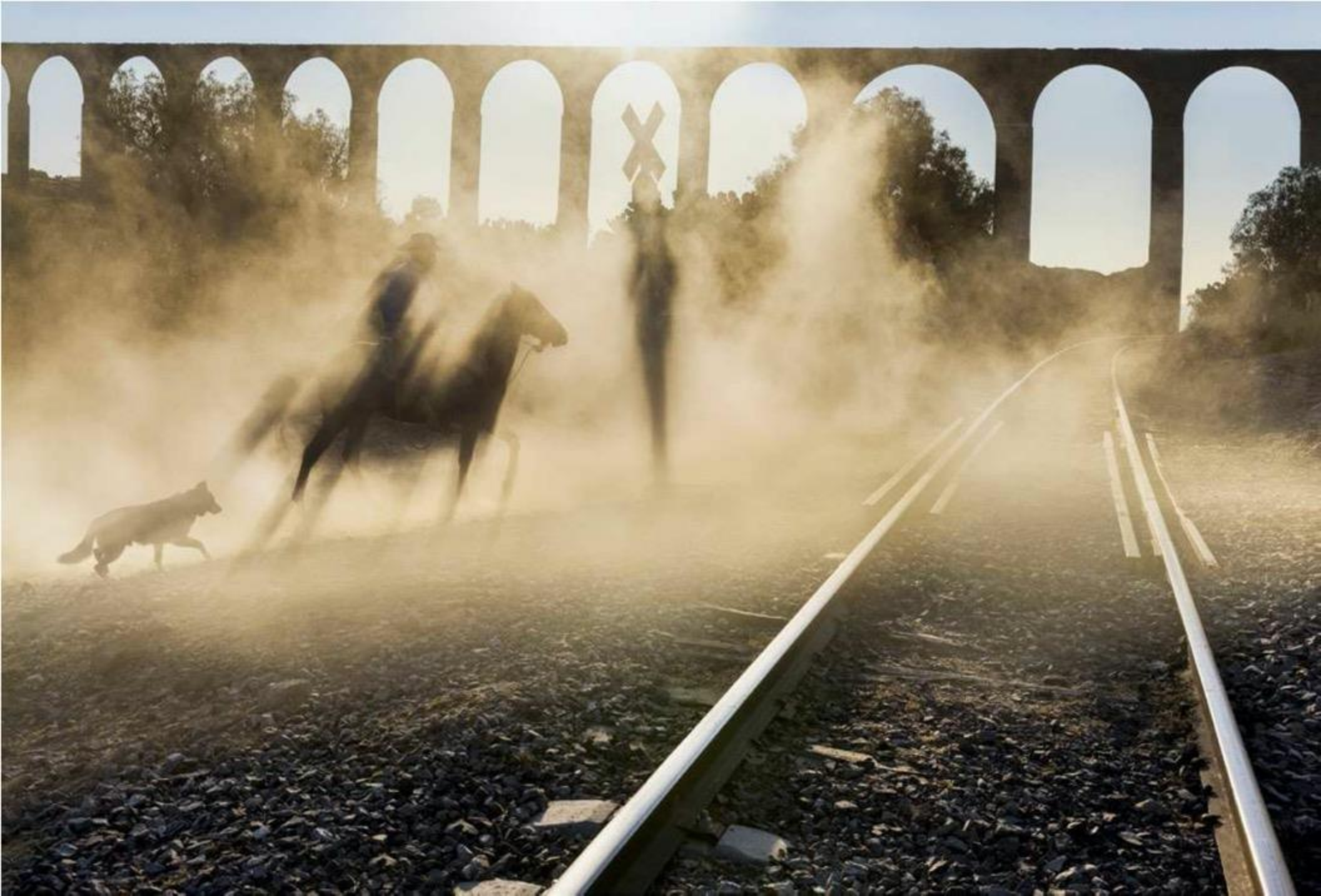
Aqueduct of Padre Tembleque | MEXICO-10082
